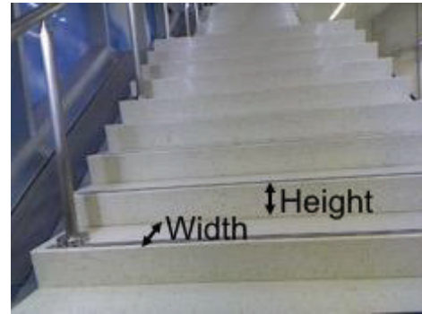
(b) The definition of stair width and height in a typical stair.
